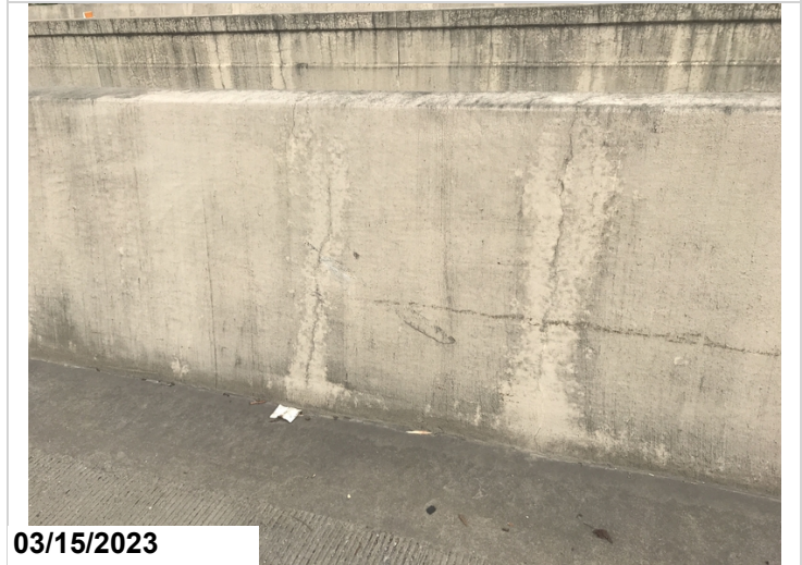
Span 3 Right cracking
