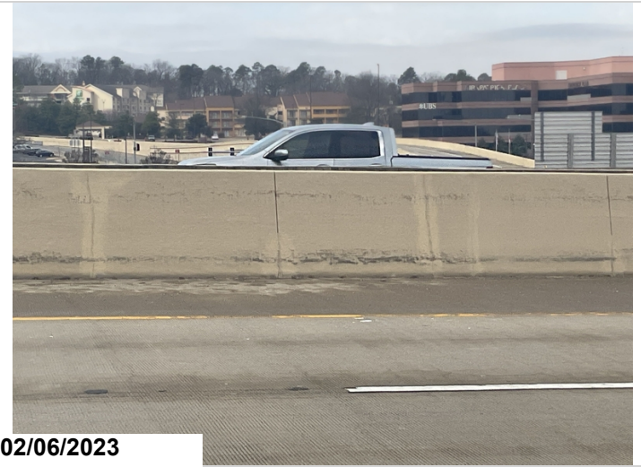
Right bridge rail vertical cracking common left bridge rail.
