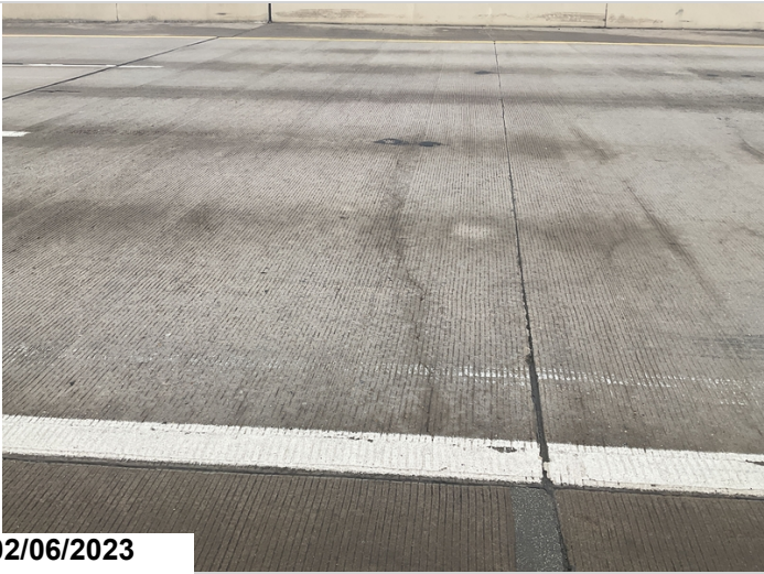
South approach slab transverse cracks.
