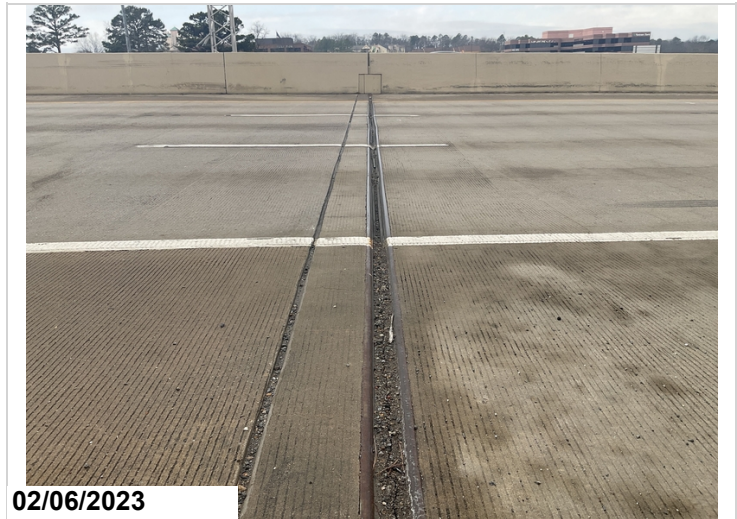
Bent 1 joint seal full of debris.
