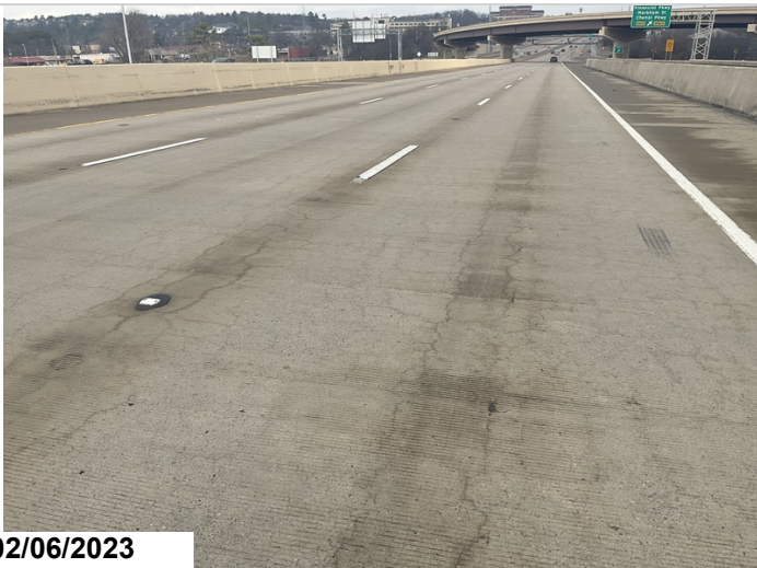
Longitudinal cracks in the deck over the top flange of beams.
