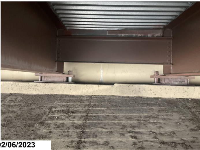
Bent 1 vertical crack with efflorescence.
