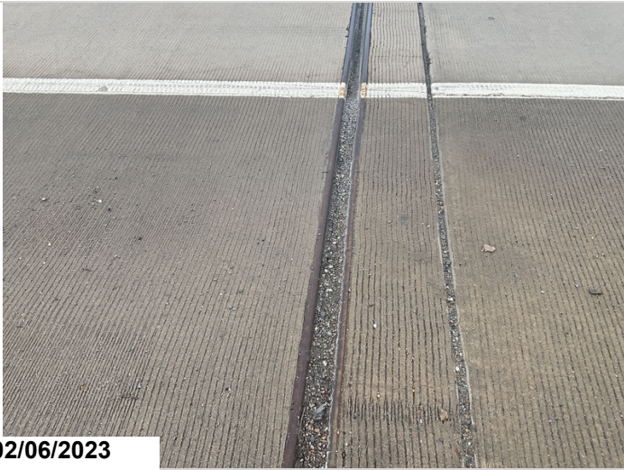
Bent 5 debris impact to joint seal. Common bent 1.
